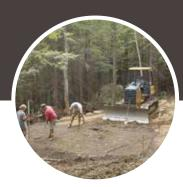
It is best practice to install a gravel pad no matter what your foundation type is. This type of preparation encourages proper drainage.
