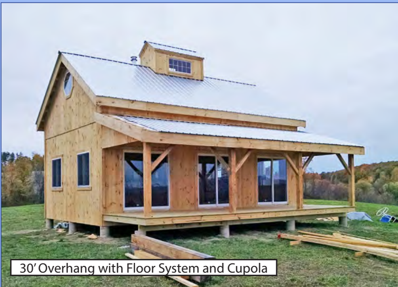
30' Overhang with Floor System
